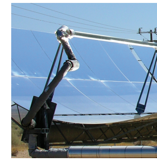
Parabolic Solar Trough
